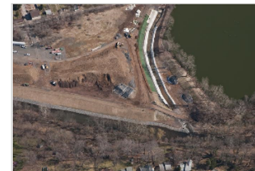
A 2010 aerial view of the BoRit asbestos site following two phases of removal action. Photo by: salbocutti.com
